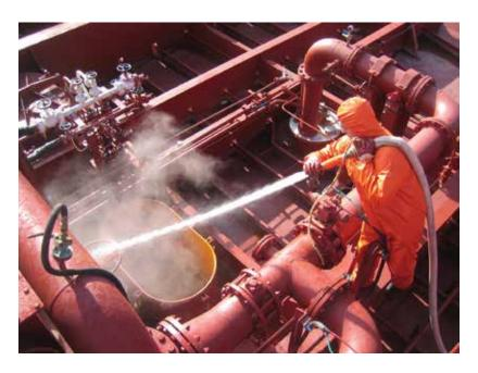
In today's safety conscious work place, the preferred option is of no-man entry into a confined space; accordingly Dovewell has developed a range of technologies and methods using tank cleaning heads, vacuum transfer systems and other pumping solutions to clean tanks and vessels either remotely or with minimum man entry.
